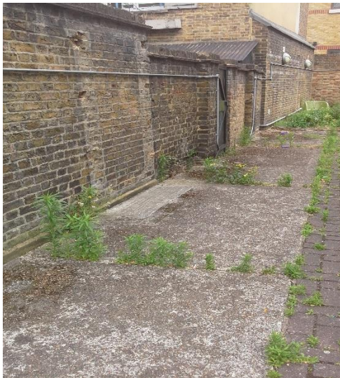
Evidence: footpath leading Sheffield House to Marcus and Bryanston House
