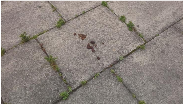
Evidence: Dog fouling and weeds in Lambeth
