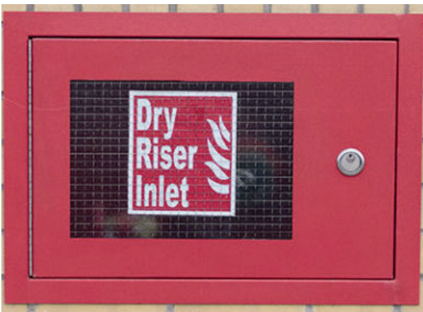
Dry riser in every building for emergency services
