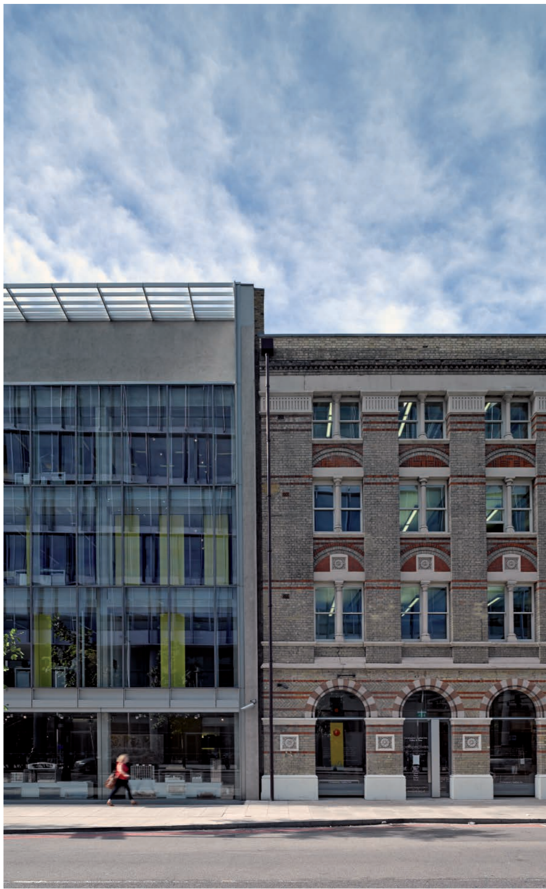
Allies and Morrison Studios, Southwark St, SE1
