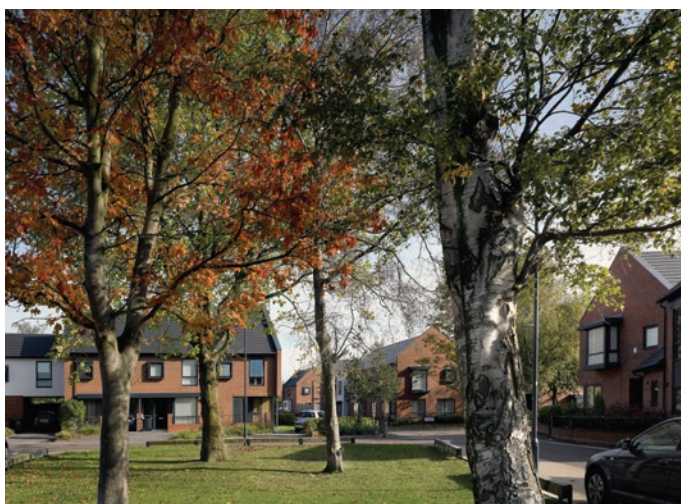
An example of Family homes fit for the future in Warburton Hey, Rainhill, a project from DK-A and Torus Housing Association.
